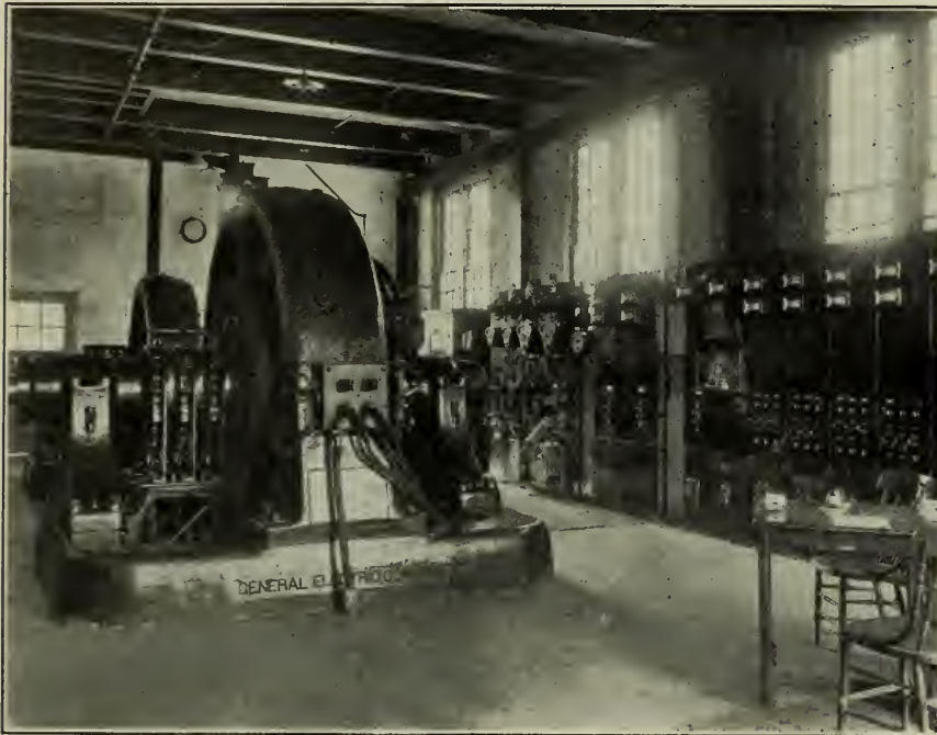
MAIN FLOOR IN TRANSFORMER STATION
